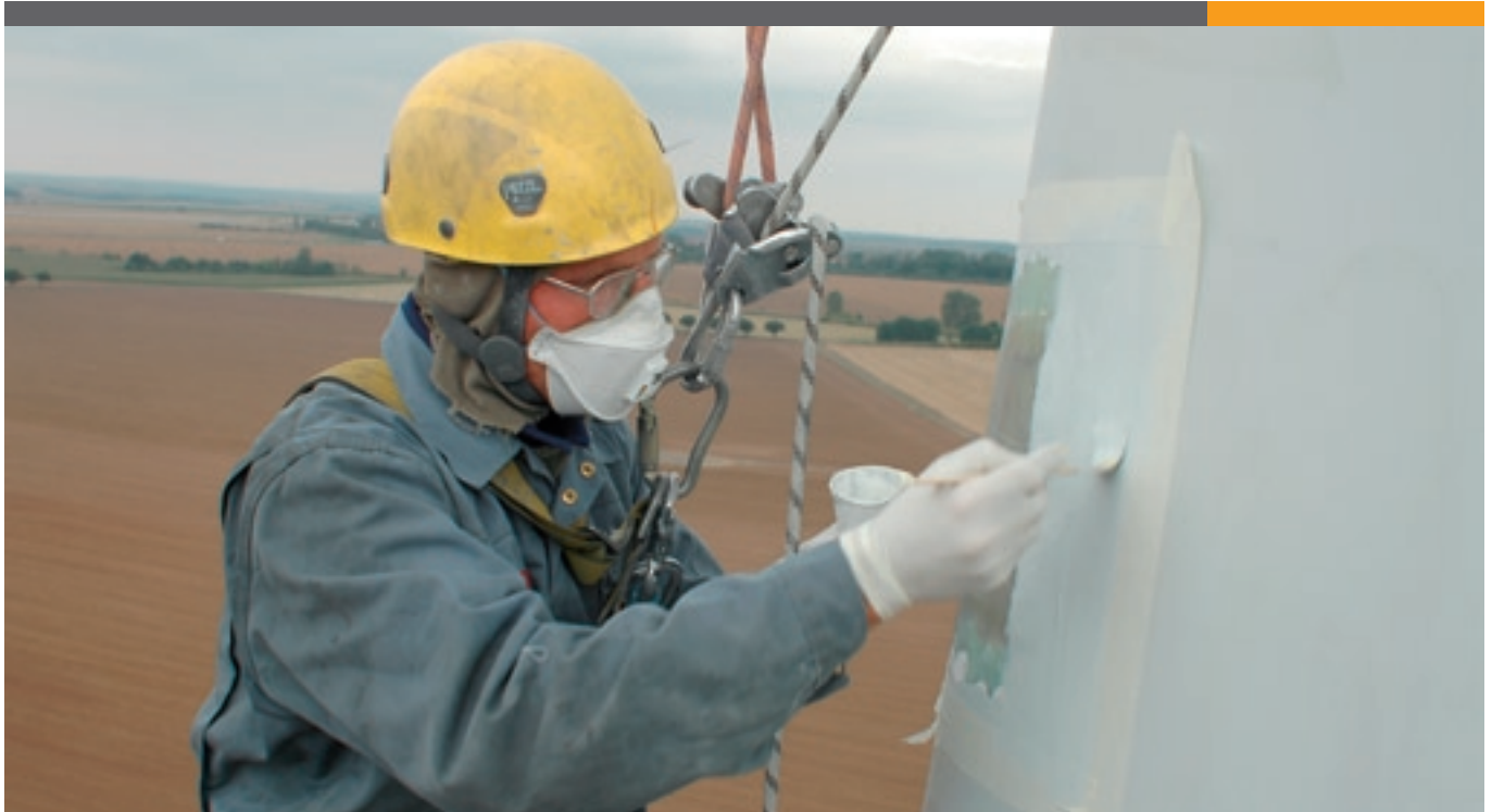
Repair of a rotor blade on site
